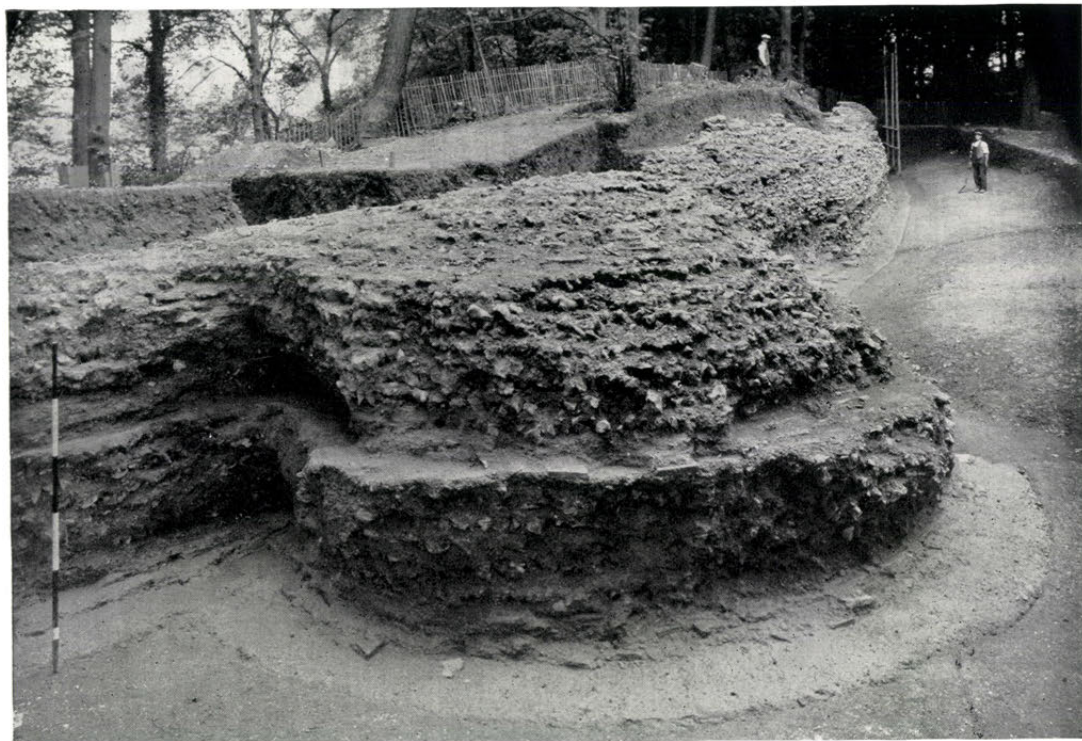
A. Second-century wall-tower at south corner : exterior
