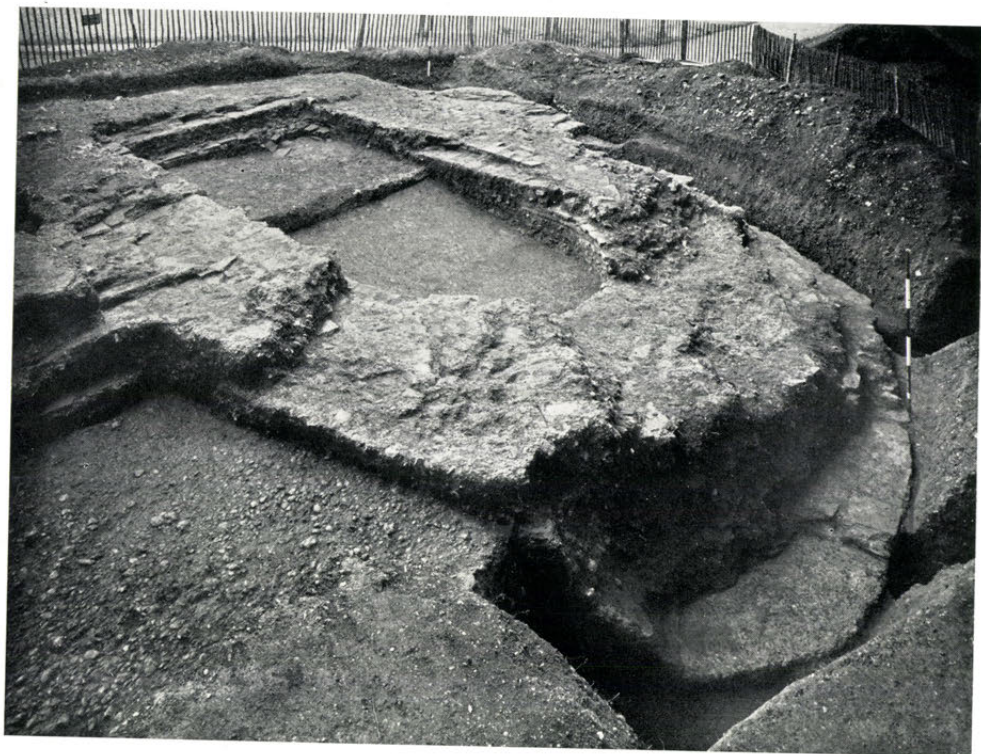
A. The foundations of the north-east tower of the south-east gate, showing the metalling of the earlier Watling Street in the left foreground. ( See p. 65 )
