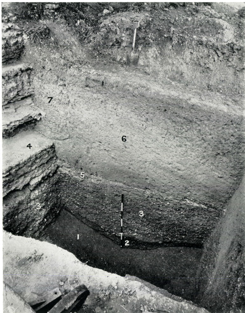
Section G-H (compare fig. 3, and pl. CXIX). 1, the ditch ('The Fosse') of the first Roman city; 2, the silt in the ditch; 3, the material of the early Roman bank thrown back into the ditch to form a basis for 4, the defensive wall of the second Roman city. 5 is the mortar-spread at the building-level of the wall. 6 is the bank contemporary with the wall, and 7 is the trench dug probably in the eleventh century by tile-robbers. (See p. 53)
