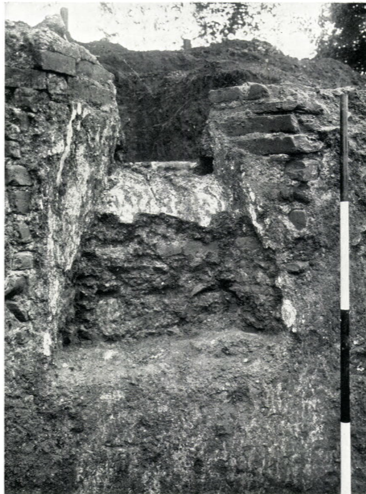
B. After removal of Roman blocking. ( See fig. 6 and p. 79 )
