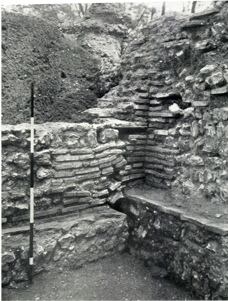
A. Wall-tower 228 feet south-west of south-east gate : junction between tower-wall and city-wall on inner side, showing subsidence and levelling during construction. ( See p. 59 )
