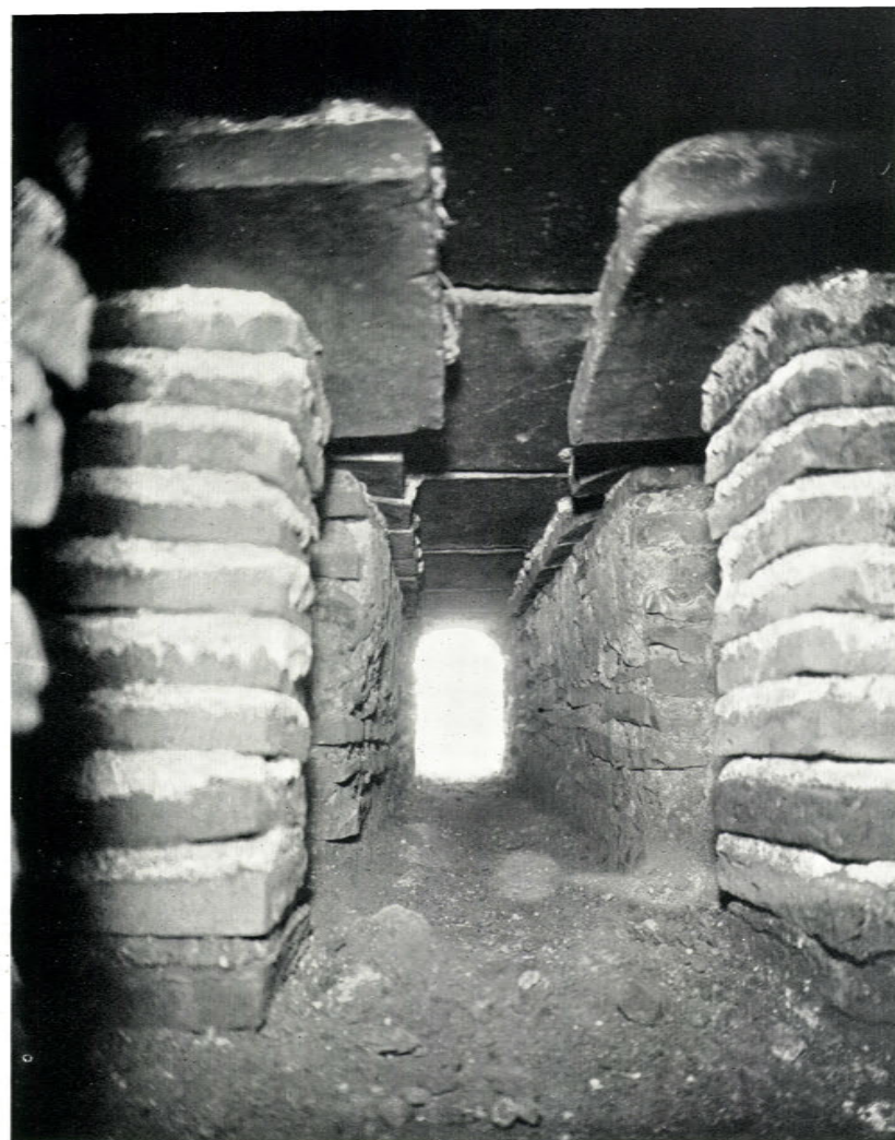
B. Flashlight photograph taken beneath the floor of room 7, showing furnace-flue in distance and pilae 2\frac{1}{2} feet high in foreground
